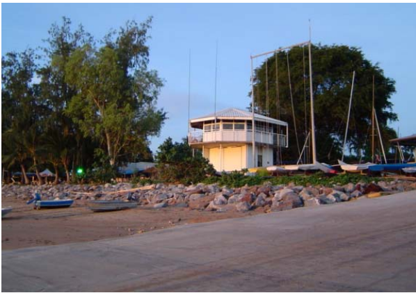
New DSC boat ramp with race tower in background
